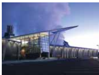
Hellisheiði Power Plant. Photo: Almar Sigurðsson.
