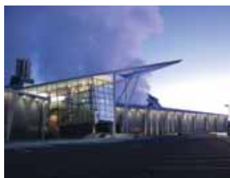
Hellisheiði Power Plant. Photo: Almar Sigurðsson.
