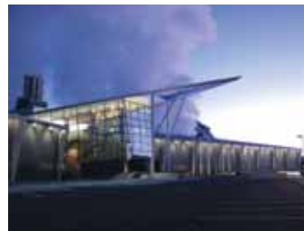
Hellisheiði Power Plant. Photo: Almar Sigurðsson.
