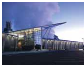
Hellisheiði Power Plant. Photo: Almar Sigurðsson.
