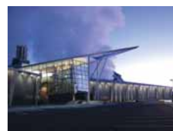
Hellisheidi Power Plant. Photo: Almar Sigurdsson.
