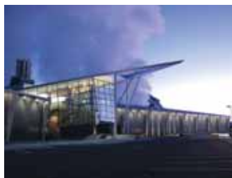
Hellisheidi Power Plant. Photo: Almar Sigurðsson.
